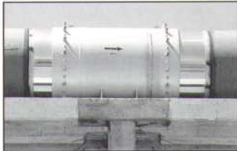
Installation of one of the 54" Dble. TP2 Expansion Joints pictured at left. This Refinery has 34 other TP2's installed.
